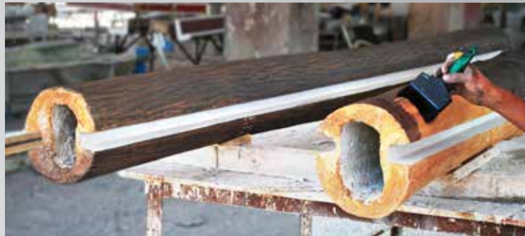
10 The post halves are assembled to form a single hollow column. A channel guide is pre-fabricated into the columns to accommodate the GFRG panels. Stain is applied to reveal the detail of the Banyan tree bark.
