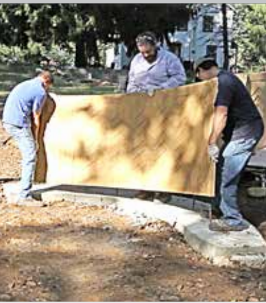
8 Precast panels are placed onto footers and fastened using anchors and rebar.
