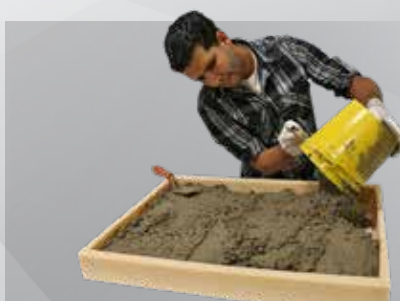
6 CONCRETE IS POURED INTO PREPARED MOLD OF PLAQUE
