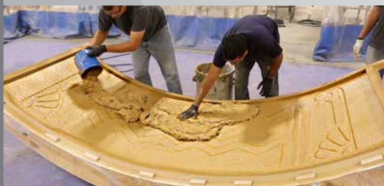
6 The GFRC backer mix (with AR glass fiber) is then applied.
