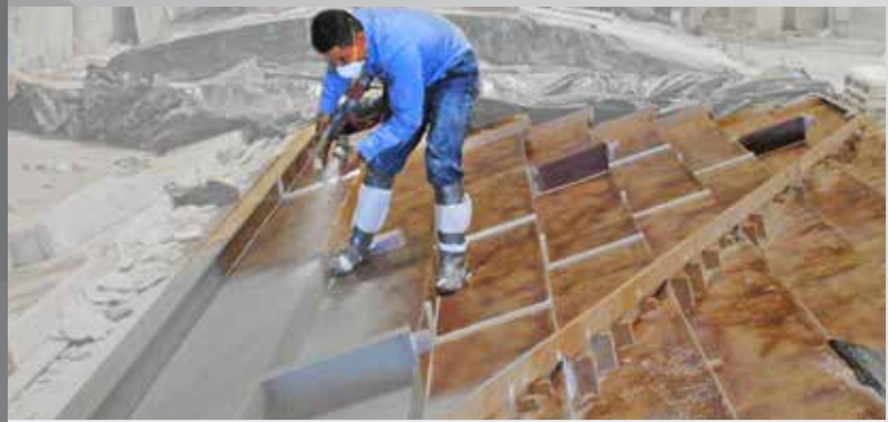
1 Two layers of a Forton™ VF-774 enhanced GFRC face mix are sprayed over form surfaces.
