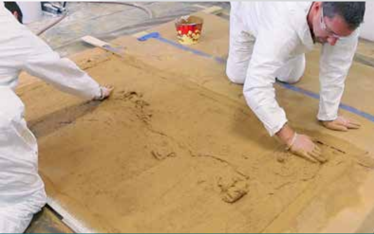
7 Back up mix (with AR glass fibers) is applied.
