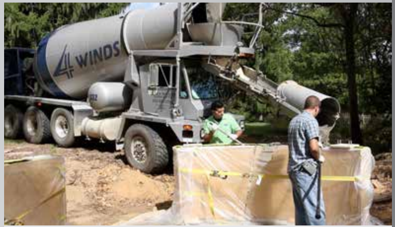
9 Ready Mixed concrete is then poured into the formwork.
