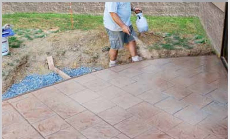
10 The concrete slab is stained and sealed.
