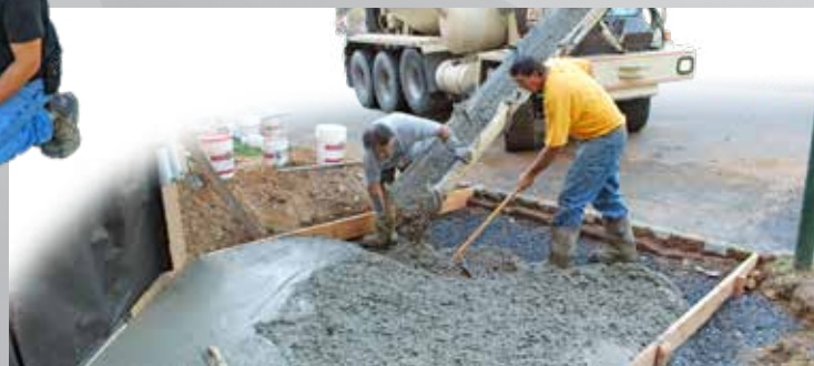
6 Ready Mixed concrete is poured at the job site.
