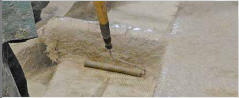
3 Compaction rollers are used to coat all glass fibers with cement slurry, remove trapped air and consolidate the composite.
