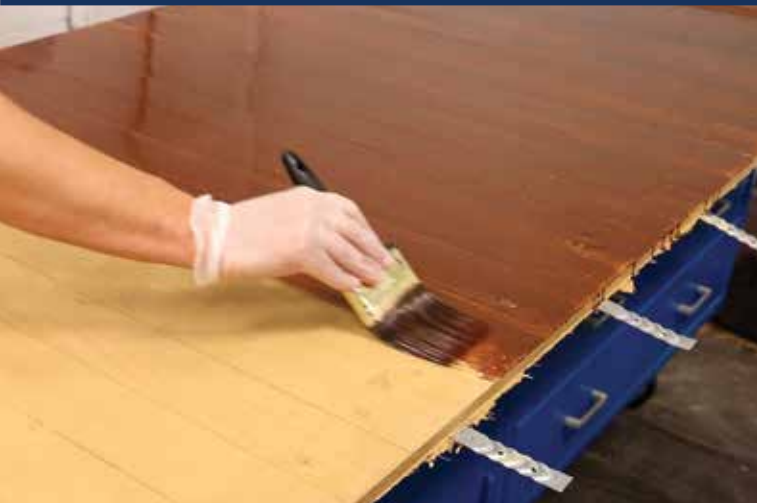
9 GFRC panels are post finished with a concrete stain and sealer.
