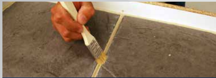
2 Textured grout is made with clay and a stiff brush.
