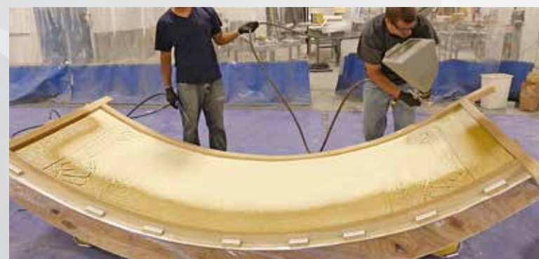
5 The GFRC face mix is sprayed using a hopper gun.
