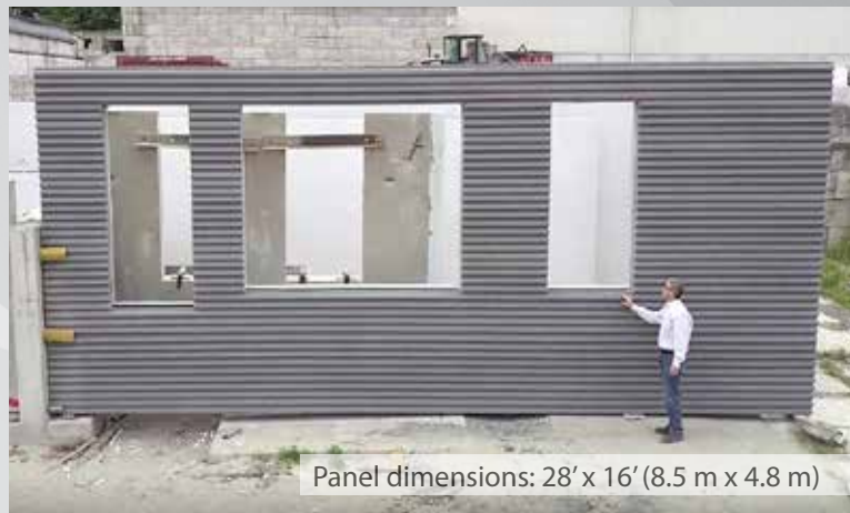
8 The panels are sandblasted and stored in Slaw Precast's yard prior to installation.
