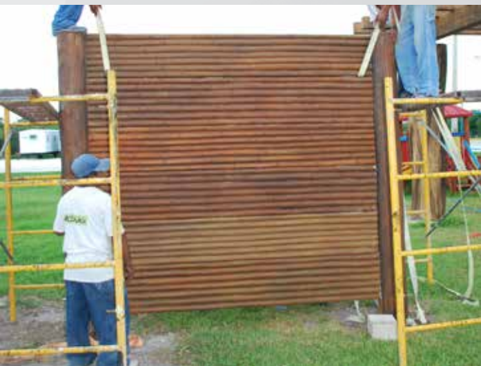
11 Columns are secured in the ground with 18" of concrete footing. Rebar reinforcement is used to marry new concrete poured into the hollow post with the footing.
