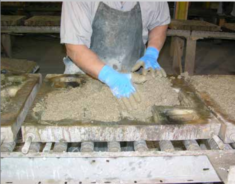
3 Concrete is then carefully cast into the mold.
