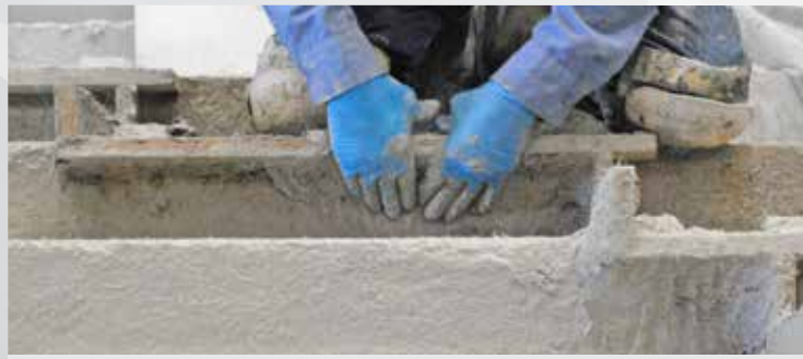
4 Additional backup mix is applied by hand to reinforce corners, edges, and reveals.
