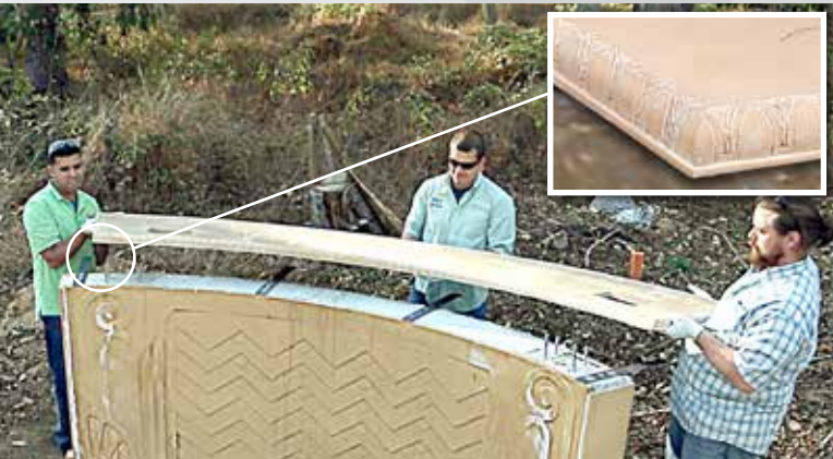
10 Custom countertops are fabricated and secured to the permanent base.
