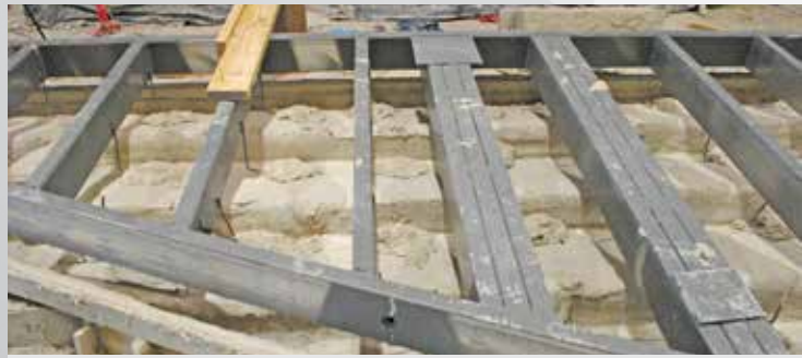
6 Pre-welded steel flex anchors attach the frame to the GFRC skin, using GFRC bonding pads.
