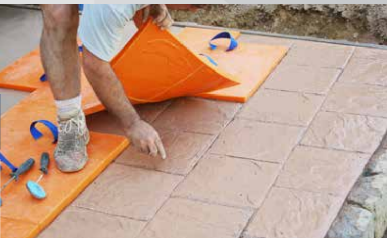
9 Stamps are then removed revealing the imprinted tile texture.
