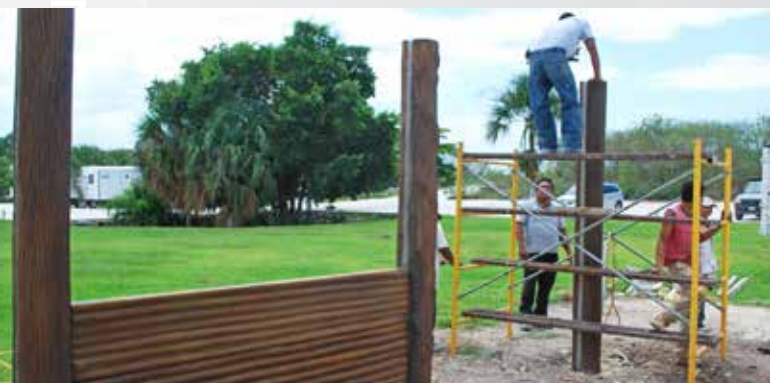
11 Columns are secured in the ground with 18" of concrete footing. Rebar reinforcement is used to marry new concrete poured into the hollow post with the footing.
